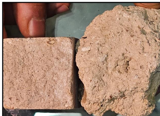
Figure 4: Comparison of old mortar (right) and modern mortar (left)
